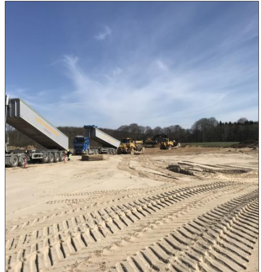
Site preparation work Compres. Station Everdrup
